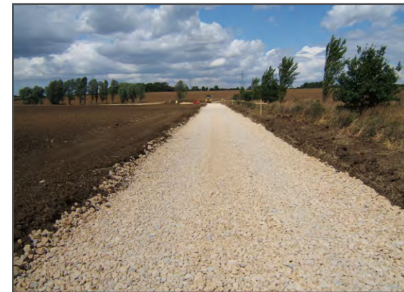
Plate 4 - Typical New Site Access Track
